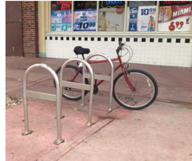
The above bicycle parking is well-spaced, properly oriented parallel to the curb, and a safe distance from the tree and the curb.
